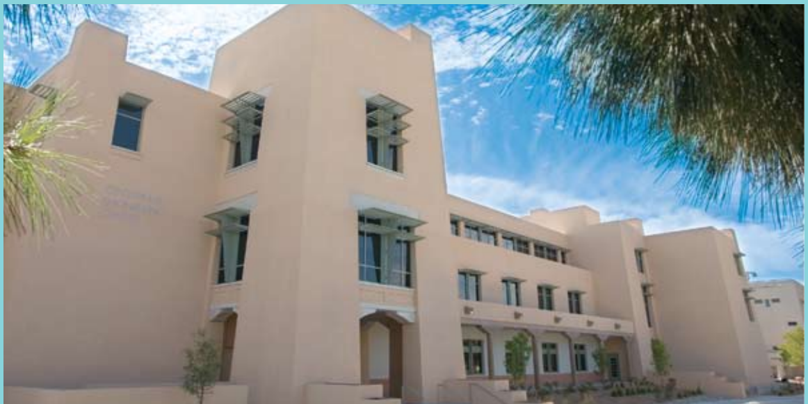
The new Centennial Engineering Center provides much-needed space for state-of-the-art engineering education and research, with classrooms, study spaces, areas for student services, and multidisciplinary teaching and research labs.
